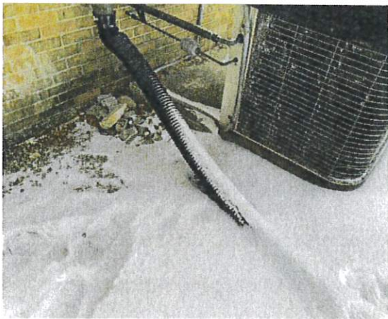
Photo 5: Roof drain location
